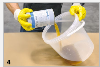
4 Transfer the mixed material into a clean, dust-free container for further processing, either by machine or manually.
