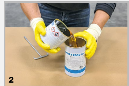
2 Pour the entire contents of hardener component A into the combination can of component B.
