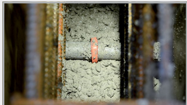
At the construction site
