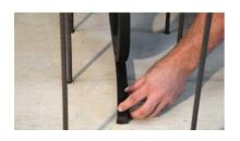
Once the swelling tape adhesive has been applied in the centre of the joint, the **MASTERSTOP bentonite swelling tape** is placed on the adhesive and gently pressed on, moving it slightly back and forth, crosswise to the longitudinal axis.
