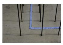
It must be ensured that the bead of **MasterMastic PU** is inside the two reinforcements with a concrete cover of 8 cm.
