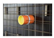
The installation of the penetration into the formwork starts after complete curing of the **MasterMastic PU** swelling paste.
