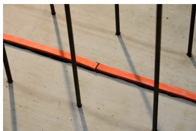
Straight butt joint
