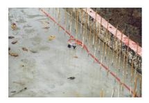
Place the hose centrally in the construction joint, within the reinforcement.
