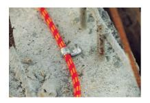
The hose can be fastened in place with metal clips for nailing (manual or nail gun).
