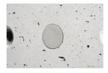
The **STOPPER maxi** must be driven in to its full depth, i.e. flush with the concrete surface.
