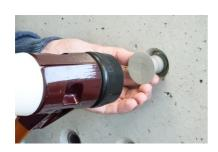
The **STOPPER maxi** is installed by driving it in with a hard rubber mallet (weight 1500 - 2000 g) using reasonable force.
