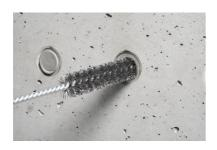
Soiled distance tubes must be thoroughly cleaned before installing the STOPPER.
