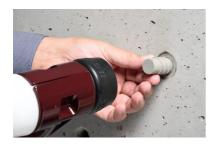
The **STOPPER in** is installed by driving it in with a hard rubber mallet (weight 1500 - 2000 g) using reasonable force.
