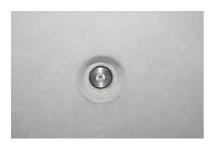
**STOPPER SCREW type in** mounted in tie point with flush seal.
