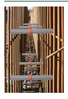
Completely installed **ActiveRings maxi**. As **ActiveRings mini/maxi** are swelling materials, appropriate measures must be taken to protect them against rain until concreting.
