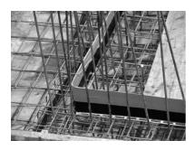
Fix the element's support rail using a tie wire.
