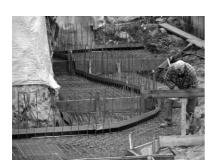
The **MASTER joint sheet metal** elements can be bent in any way.
