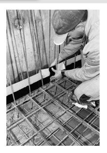
Place the **MASTER joint sheet metal** element in the centre of the rising wall on top of the upper reinforcement layer.
