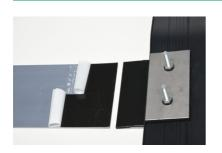
The protective foil of the joint sheet metal to be connected must also be removed.
