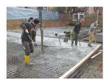
Before the segment is concreted, the protective foil must be removed from the joint sheet metal.
