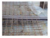
The **stopend panel joint sheet metal ABS** is positioned between the lower and upper reinforcement layer (foundation – foundation area) or the outer and inner reinforcement layer (wall – wall area). The perforated plate is fastened to the reinforcement using binding wire.
