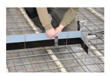
The **VB joint sheet metal** must overlap by at least 6 cm in the area of the joint, in the straight sections and also in the corner area.
