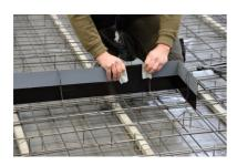
Overlap the **VB joint sheet metal** by <u>at least 6 cm</u> and press the two ends firmly together. The joint must be glued over its full height and entire surface to prevent subsequent water permeation. There must be no contamination on the adhesive surfaces that could interfere with bonding.
