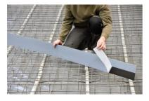
Remove the bottom half of the parted protective foil from the special coating.
