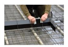
Overlap the **VB joint sheet metal** by <u>at least 6 cm</u> and press the two ends firmly together. The joint must be glued over its full height and entire surface to prevent subsequent water permeation. There must be no contamination on the adhesive surfaces that could interfere with bonding.
