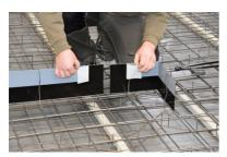
To do so, the upper protective foil must be turned back in the area subsequently to be joined.
