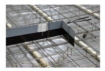
Secure the joint with one of the fixing clips provided and fold the protective foil back onto the special coating.
