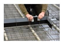
Overlap the **VB joint sheet metal** by <u>at least 6 cm</u> and press the two ends firmly together.
