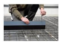
Place the **VB joint sheet metal** in the centre of the rising wall on top of the upper reinforcement layer. Push the mounting brackets with a maximum distance of 70 cm over the sheet metal and fix them to the upper reinforcement layer with binding wire.
