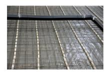
Prepared joints in the straight sections as well as the corner area.
