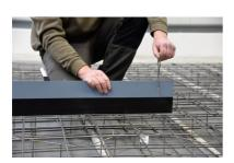
Place the **VB joint sheet metal** in the centre of the rising wall on top of the upper reinforcement layer.
