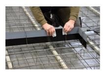
Overlap the **VB joint sheet metal** by <u>at least 6 cm</u> and press the two ends firmly together.
