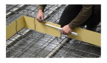
The joint of the **Joint sheet metal MB Overlap** can be made without glue, only by overlapping the two ends.
