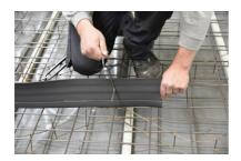
**MASTER-MultiFlex (MMF 140)** is placed on the upper reinforcement layer in the centre of the rising wall. Place the mounting brackets (2 pcs/m), over the joint tape and fix them with binding wire to the upper reinforcement layer.
