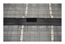
Apply the MMF 140 adhesive tape on the prepared surface. Remove the backing before bonding with the crack-inducing profile.
