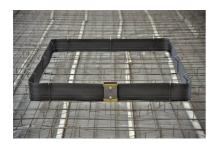
Secured joint tape with MMF 140 MASTER-Connect "active"
