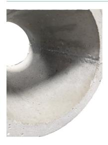
Smooth out the joints inside the casing to obtain a clean surface for the possible installation of an gasket insert or similar.
