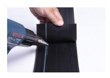
A hot air gun is used to weld the joint tapes together, one below
