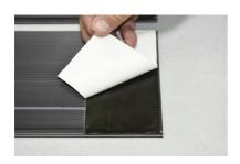
Apply the **MMF 140 adhesive tape** (width 75 mm), from the **MMF**
