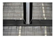
Bond the crack-inducing profile with the prepared surface of **MASTER-MultiFlex (MMF 140)** on the water-facing side.
