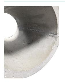
Smooth out the joints inside the casing to obtain a clean surface for the possible installation of an gasket insert or similar.
