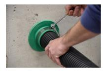
Secure the pipe by hand-tightening the clamp.
