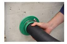
Then place the clamp over the connection seal and push the media pipe in as fas as it reaches the stop.
