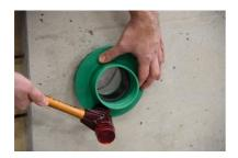
Drive the **Connector connection seal** in evenly with a rubber or plastic mallet until the gasket is flush against the component surface.
