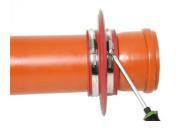
Apply lubricant to the clamping range of the strap, then tighten the clamping straps sufficiently using a screwdriver to prevent the **RONDO Protect sealing collar** from shifting.
