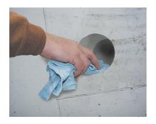
Before installing the **MASTER-SEAL** modular seal, the inside of the core drill hole and the outside of the gas, water, sewage pipes as well as the cables have to be cleaned.
