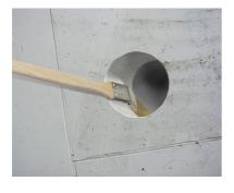
When installing a **MASTER-RING** gasket insert in a core drill hole the inside of the core drill hole has to be preserved with an epoxy resin ( PROTECT EP resin). The preservation serves to obtain a smooth surface and secondly as protection of the cut reinforcement steels against corrosion.
