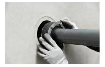
Close the gasket and reinstall the locking clip and close it as well.
