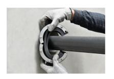
Place the **MASTER-Ring Multi split version** around the installed pipe.
