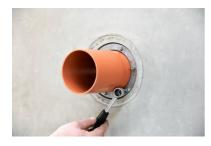
Tighten the screws crosswise through one turn. Repeat this process until all screws are tightened to the specified max. torque.
