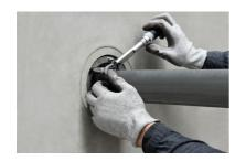
Tighten the screws to the specified max. torque. (Ø 100/150/200 = 5Nm; Ø250 = 10Nm).
