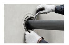
Tighten the screws crosswise through one turn.
