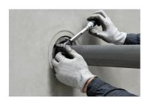
Tighten the screws to the specified max. torque. ( $\emptyset$  100/150/200 = 5Nm;  $\emptyset$ 250 = 10Nm).
