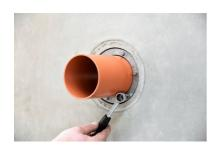
Tighten the screws crosswise through one turn. Repeat this process until all screws are tightened to the specified max. torque.
