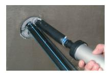
Fill the duct completely with **FLEX 2000**.
