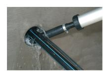
Insert the flexible nozzle into the duct and seal it with **FLEX 2000** starting from the securing block.
