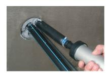
Fill the duct completely with FLEX 2000.
