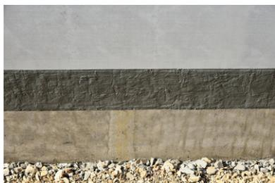
Joint horizontal/joint de construction fini, raccord radier/mur sans socle.
